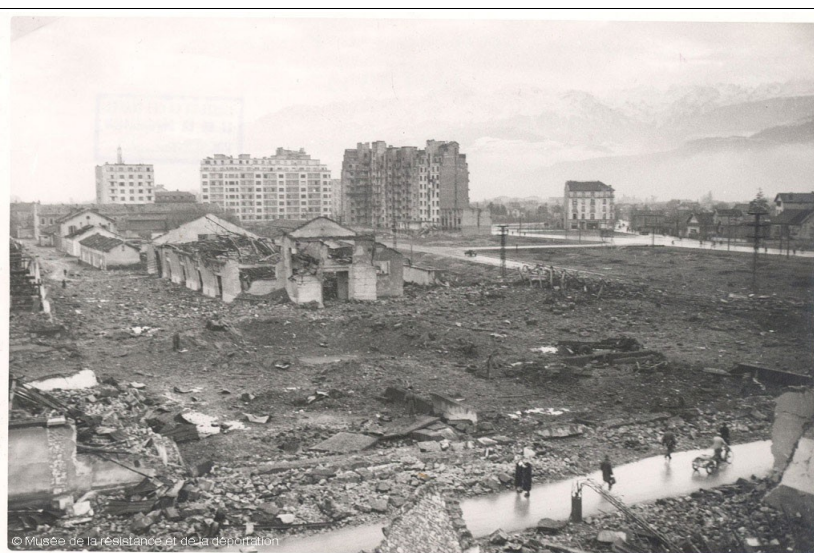
Bonne barracks after the explosion
